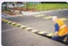
Put modules in place
