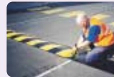
Trim rubber & clean site
