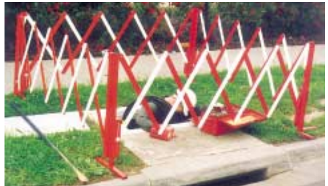
Two units used to create a safe work area
